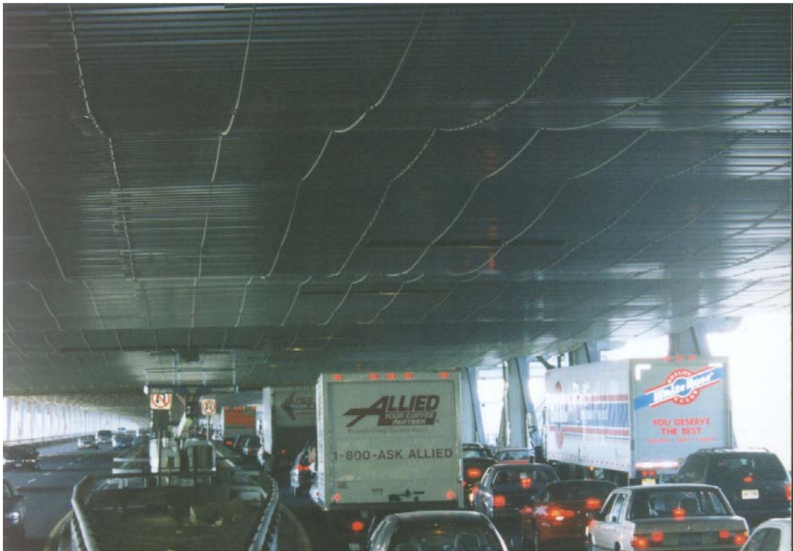
Cable Supported Platform – Looking Toward New York
