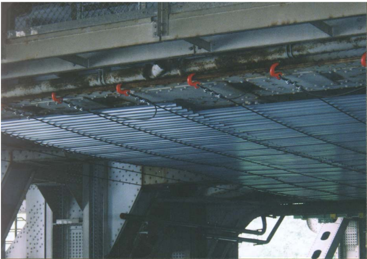
End Connection At Towers Hooks To Floor Beam
