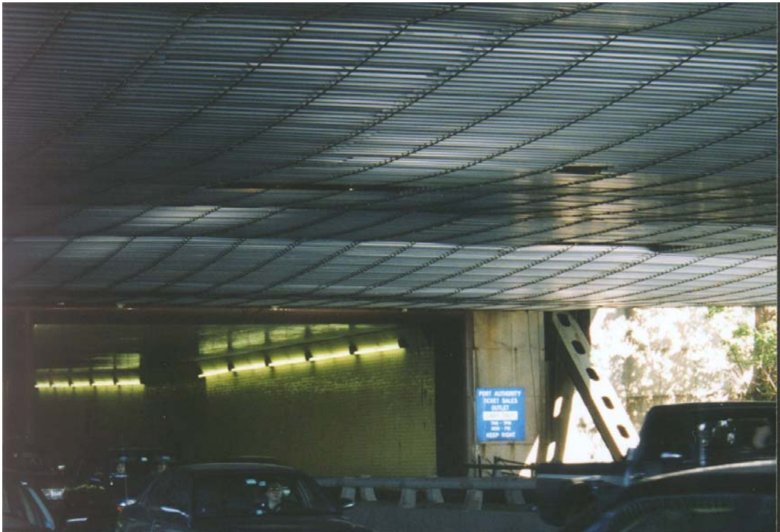
Cable Supported Platform – New Jersey Approach
