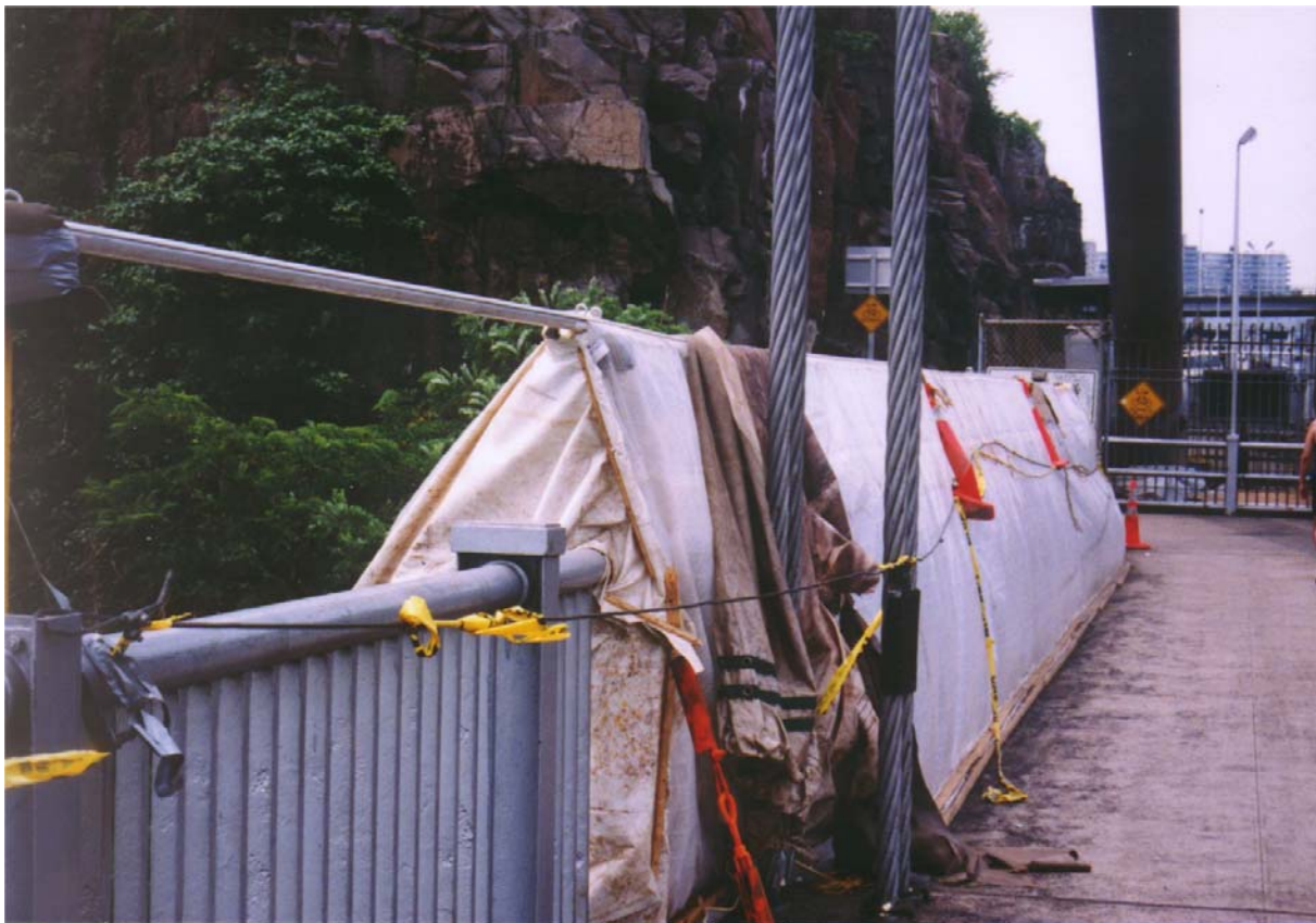
Containment Tarpaulins Over Upper Level Railing
