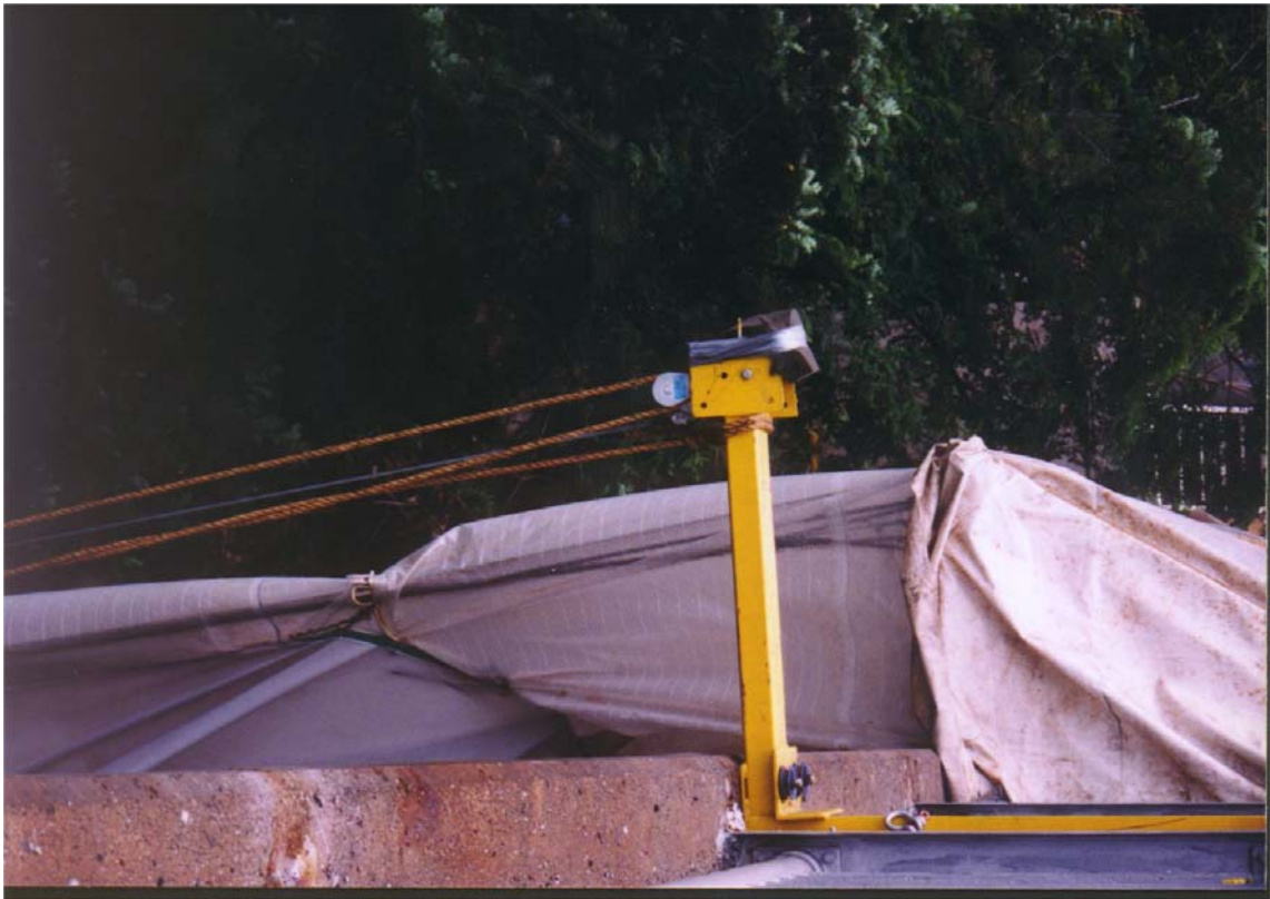
Sail System Containment Tarpaulins Pulleys & Brackets
