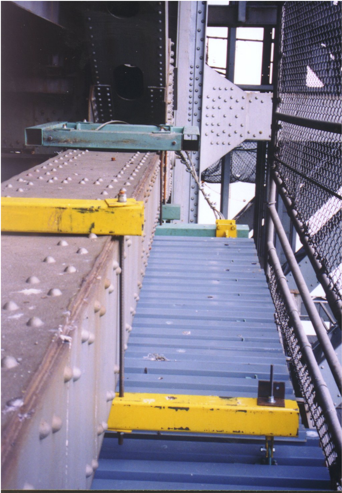
Lower Truss Chord Platform Clamping Tubes & Tie Rods Foreground (Yellow) Lower Truss Chord Platform End Clamping Support Tubes Tie Rods & Cables Background (Green)
