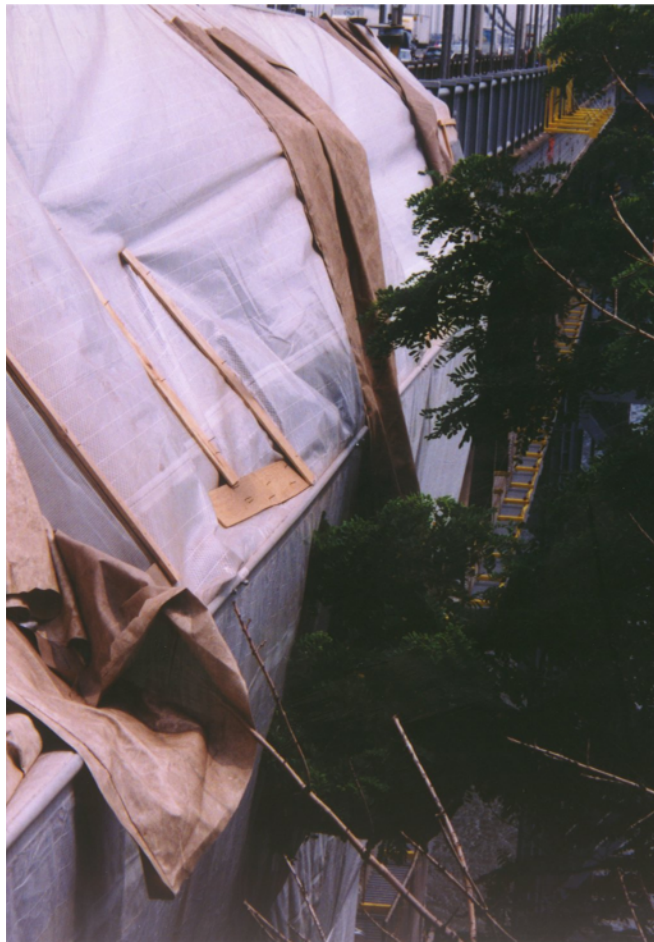
Sail System Containment Tarpaulins
