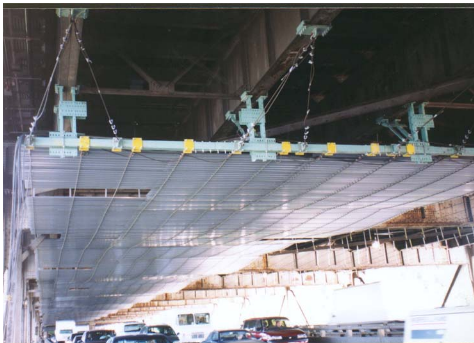
Post Brackets/Horizontal Support Beam Main Cables & Decking & Stringer Clamping Plate Tie Back
