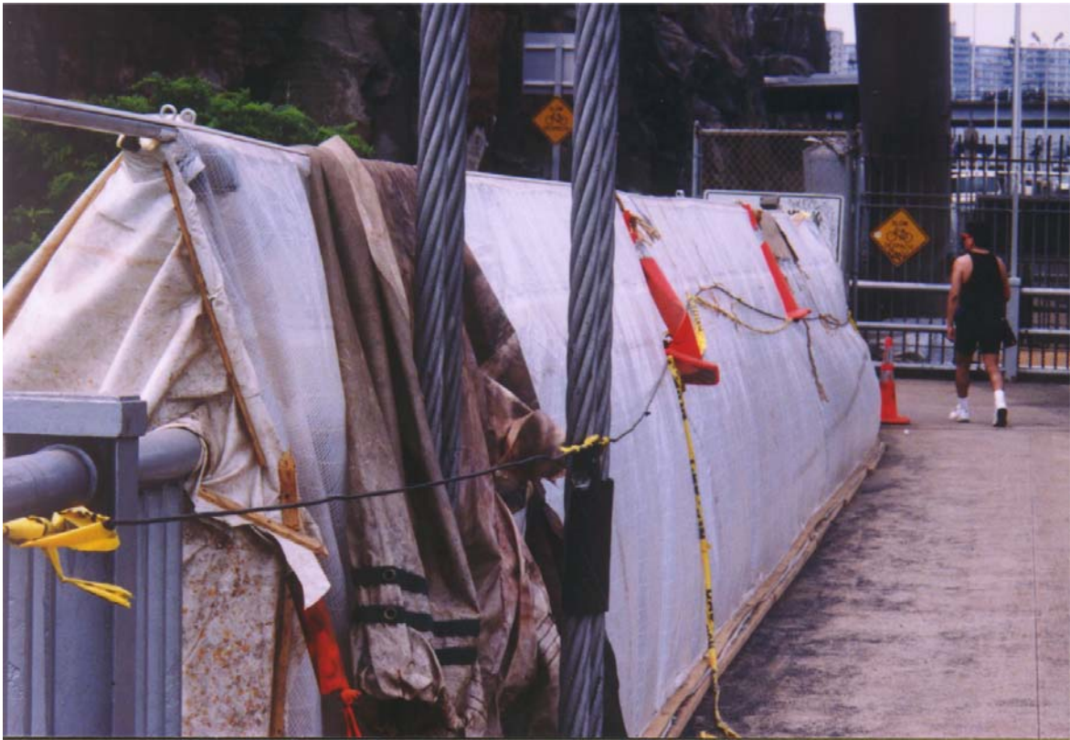
Containment Tarpaulins Over Upper Level Railing
