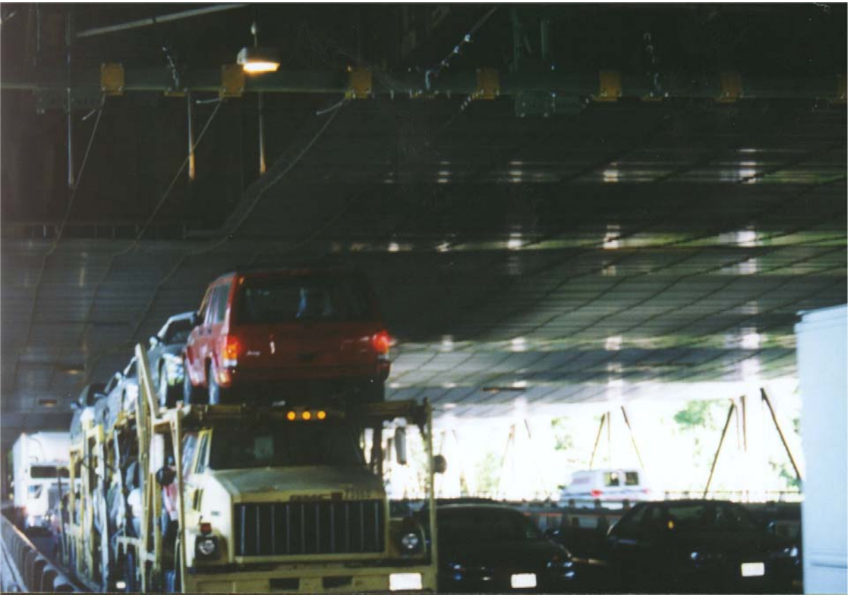
View Showing Tight Vertical Clearance
