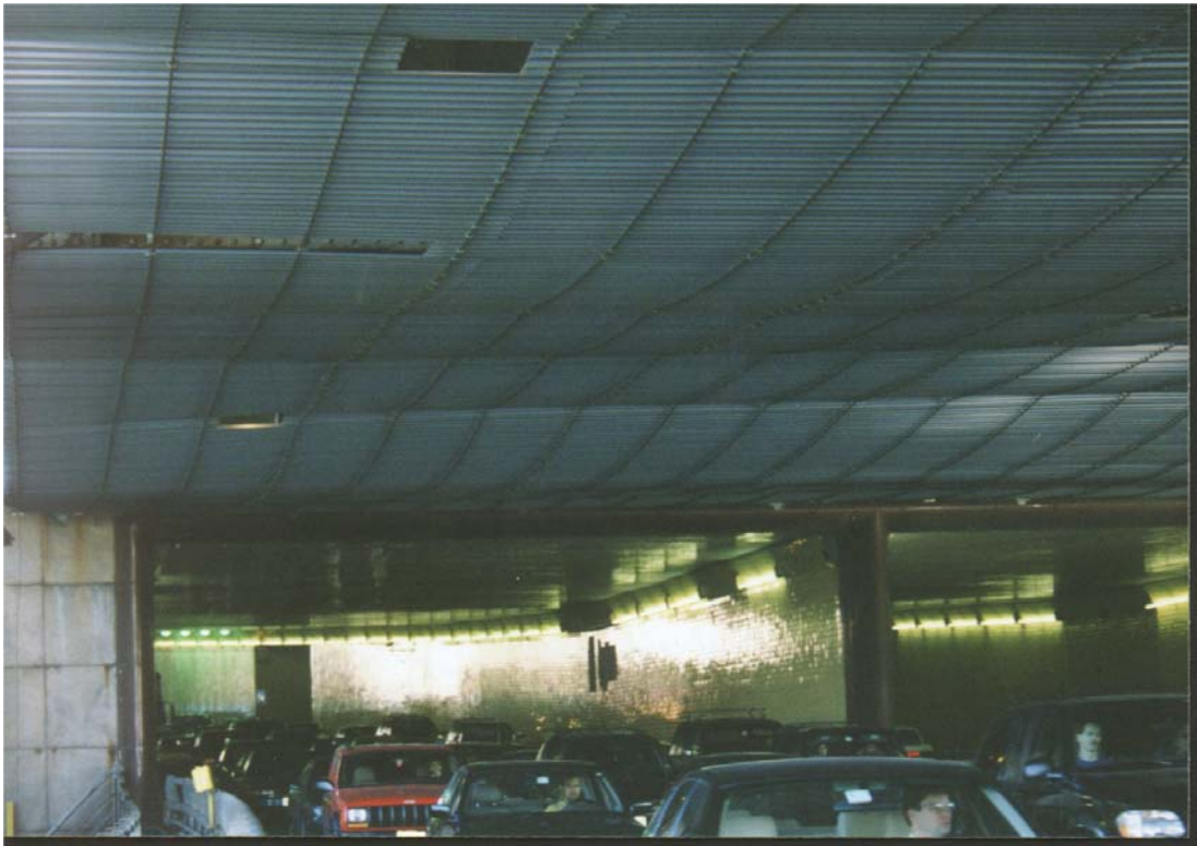
Cable Supported Platform – New Jersey Approach
