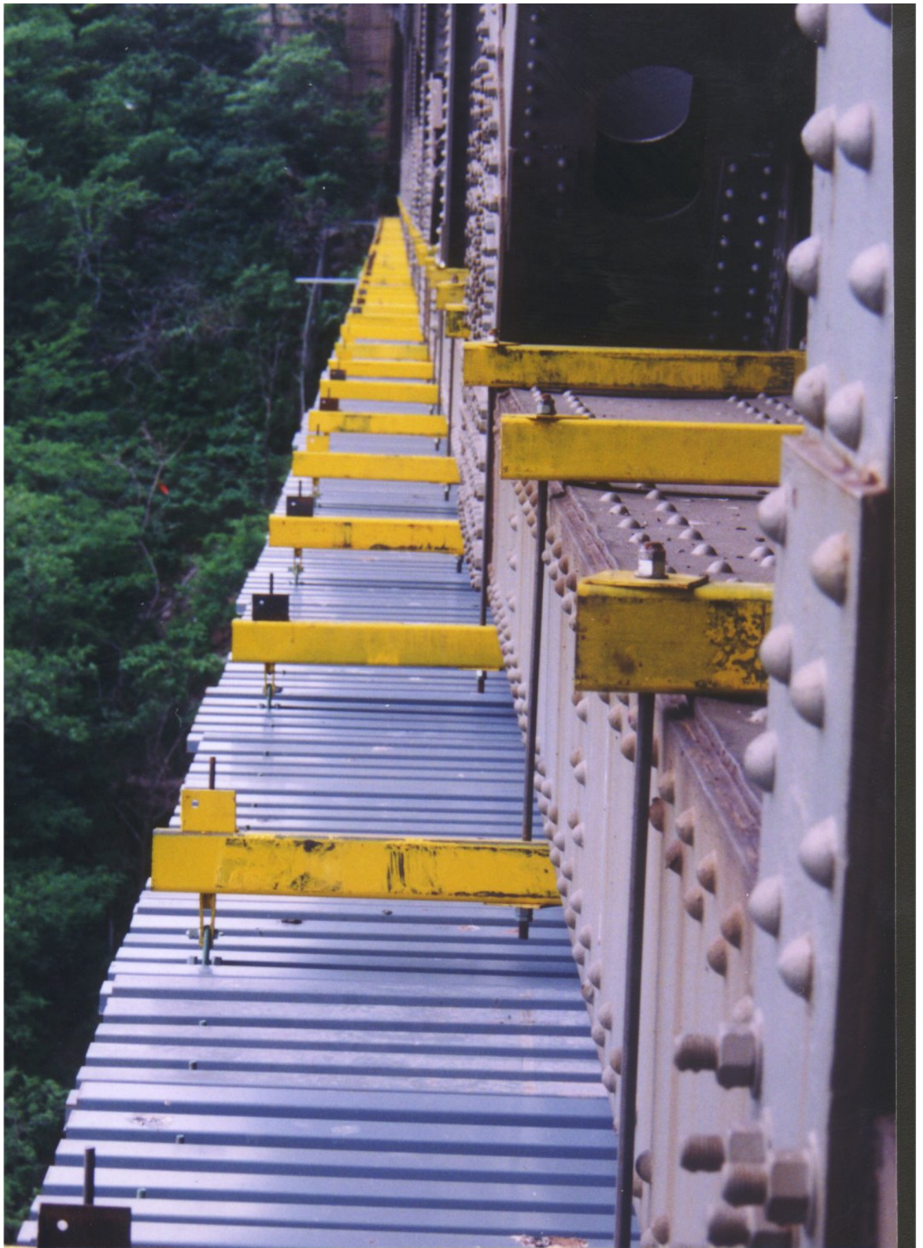
Lower Truss Chord Platform Clamping Tubes & Tie Rods
