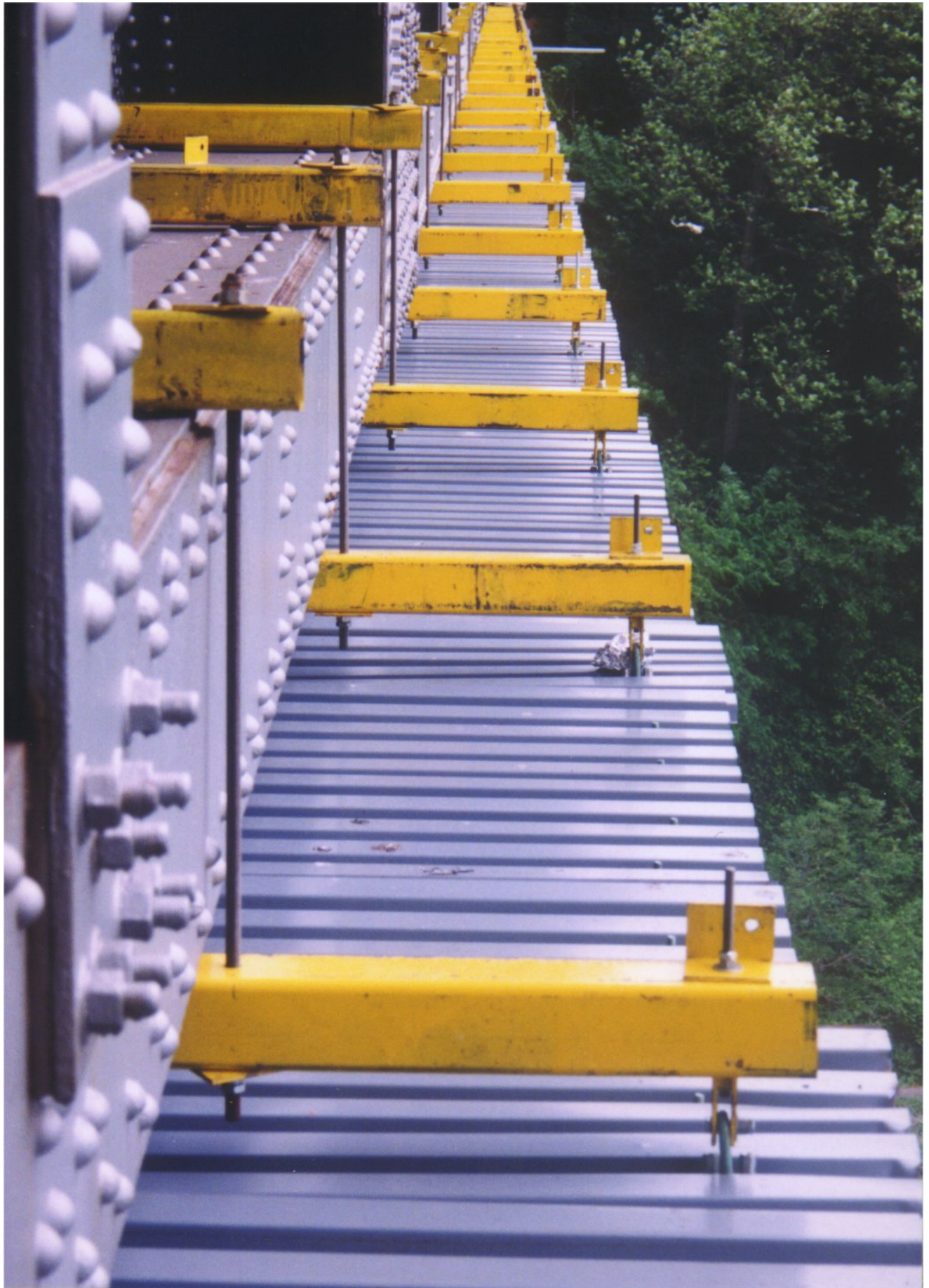
Lower Truss Chord Platform Clamping Tubes & Tie Rods
