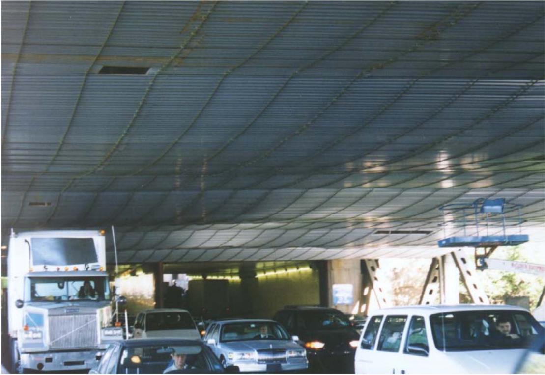
Cable Supported Platform – New Jersey Approach
